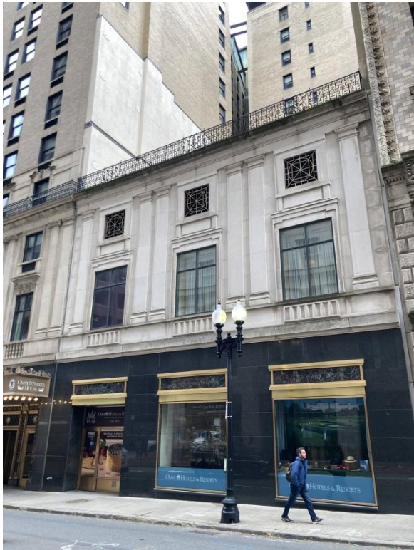
Figure 10. Tremont Street façade; south appendage. October 2021.
