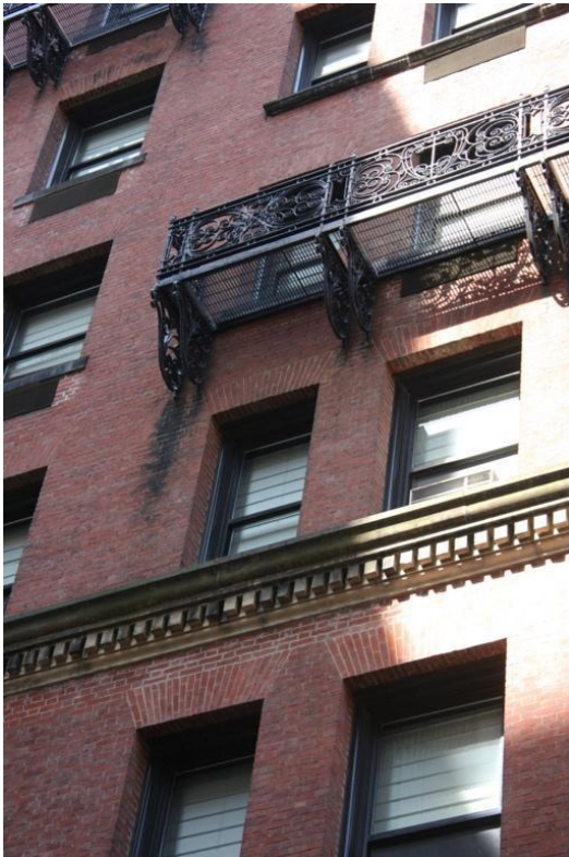
Figure 20. Parker House Annex; detail of façade. July 2020.
