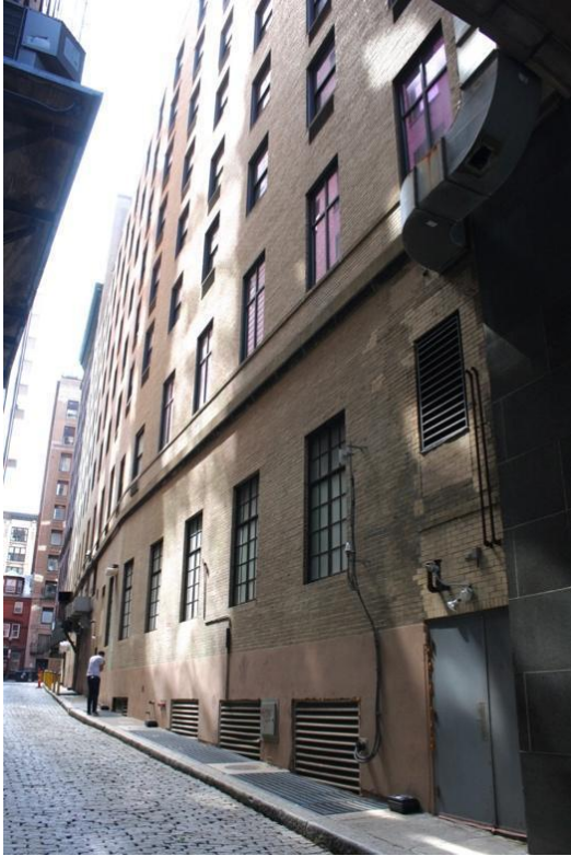
Figure 13. Chapman Place elevation, from School Street. July 2020.
