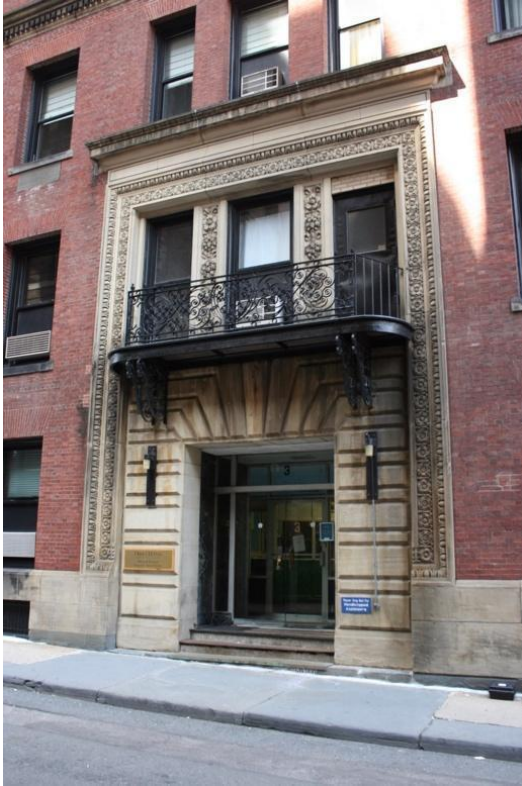
Figure 19. Parker House Annex; main entrance on Bosworth Street. July 2020.
