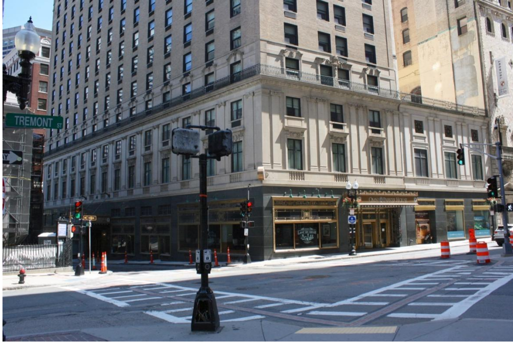
Figure 5. School and Tremont streets façades; storefronts and base. July 2020.
